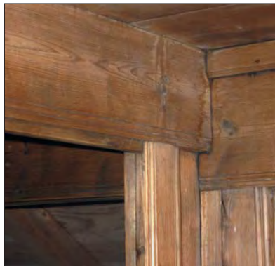
Figure 10. Decorative mouldings on beams and posts in the glasstova of the house from Múli.
