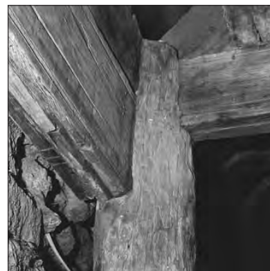
Figure 15. Post, cross beam and head beam in the dwelling room of the farm Keldur in Iceland. Note the groove from a stave wall and the decorative mouldings on the beams.
