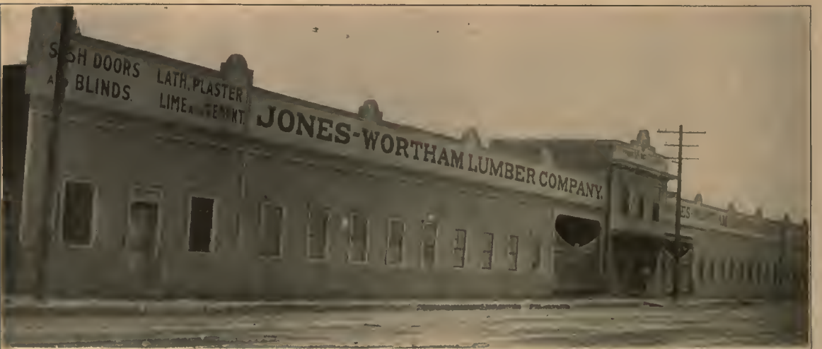
SHED OF THE JONES-WORTHAM LUMBER COMPANY, DALLAS, TEX.
