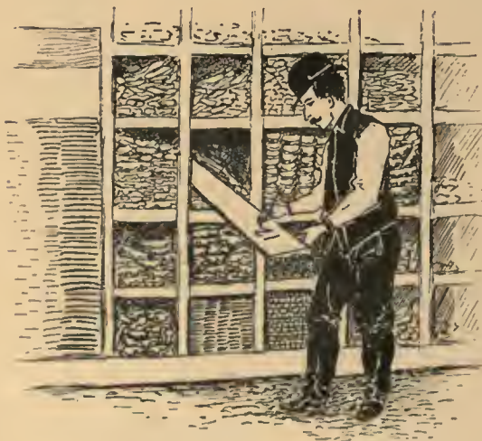
MARKING LENGTH OF MOLDING.
