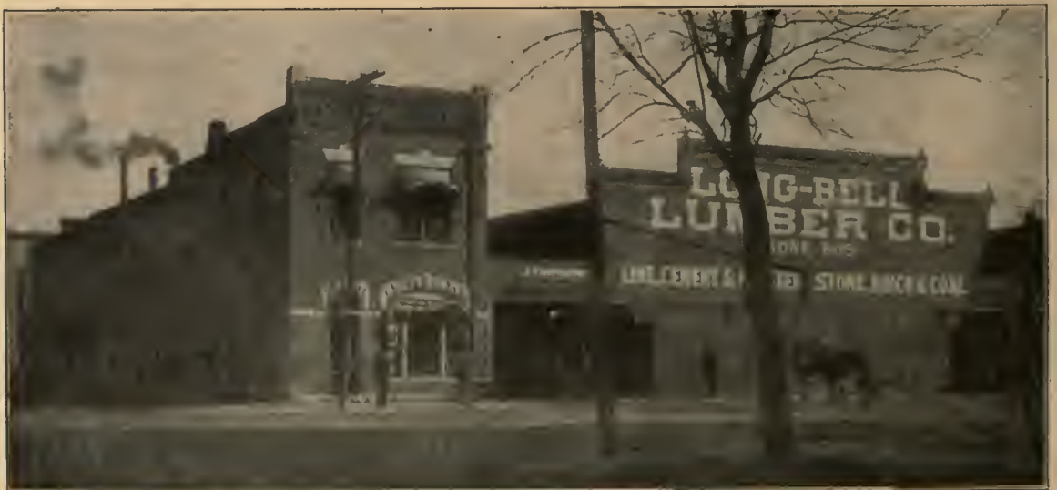
SHED OF LONG-BELL LUMBER COMPANY, WICHITA, KAN.
