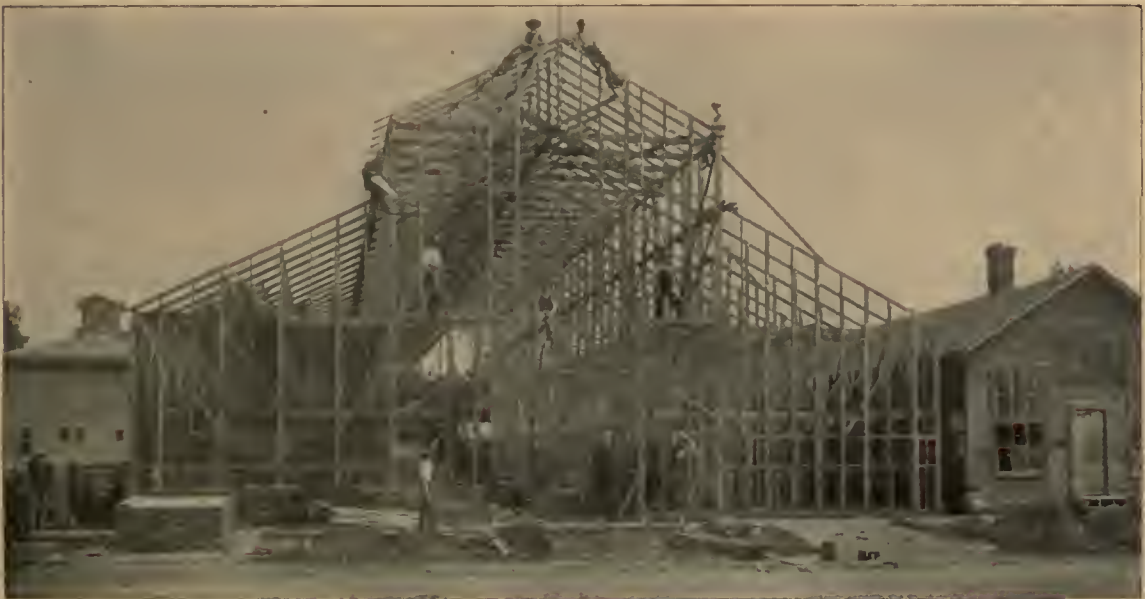
EXAMPLE XVIII--FRAMEWORK OF J. A. SMITH SHED AT OSAGE, IOWA.
