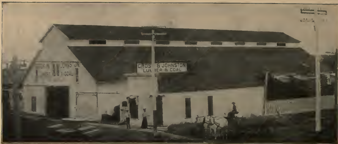
CROSS & JOHNSON'S BIG SHED AT MINDEN, NEB.
