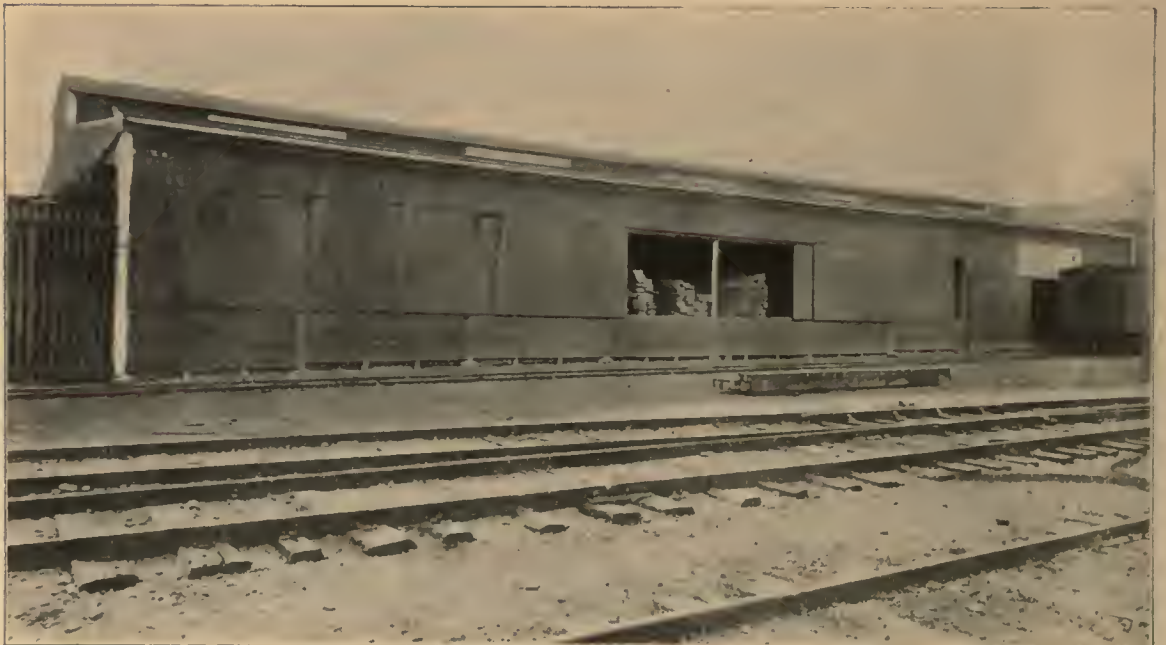
SHANNON LUMBER COMPANY'S SHED—LOADING DECK SIDE.
