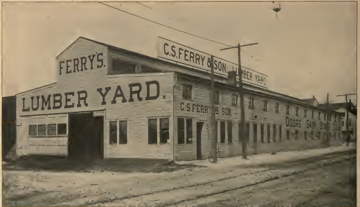
EXAMPLE XXXI—SHED OF C. S. FERRY & SON, AT PITTSFIELD, MASS.
