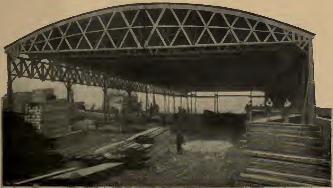
EXAMPLE XXX—MOLLOY PATENT TRUSS ROOF CONSTRUCTION.
