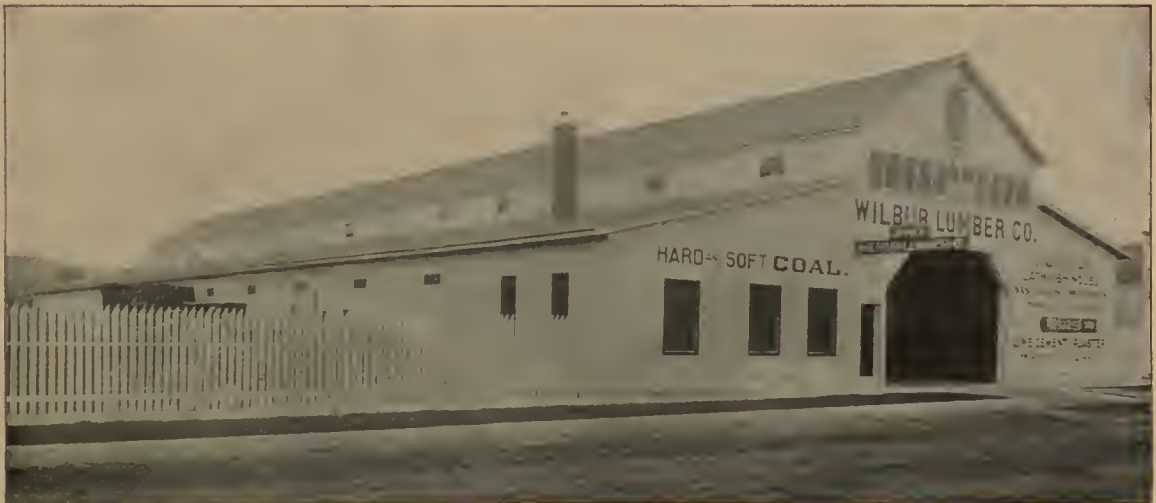
SHED OF THE WILBUR LUMBER COMPANY AT DECORAH, IOWA.
