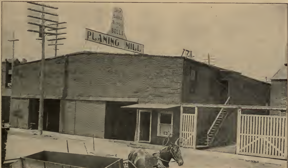
PLANT OF JOHN BELL & SONS AT PONTIAC, MICH.
