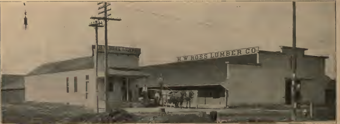
SHED OF THE H. W. ROSS LUMBER COMPANY, SIOUX FALLS, S. D.
