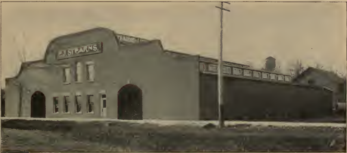
EXAMPLE XXVIII—SHED OF THE STEARNS LUMBER COMPANY, AT HUTCHINSON, MINN.
