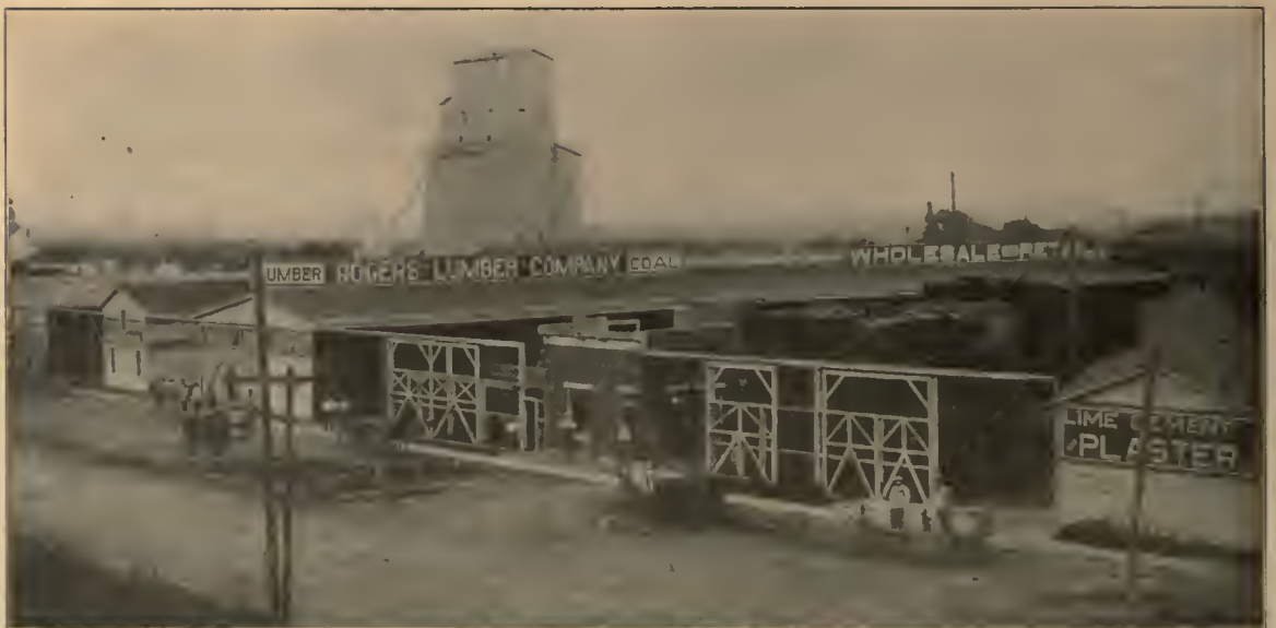
SHED OF ROGERS LUMBER COMPANY, LINCOLN, NEB.
