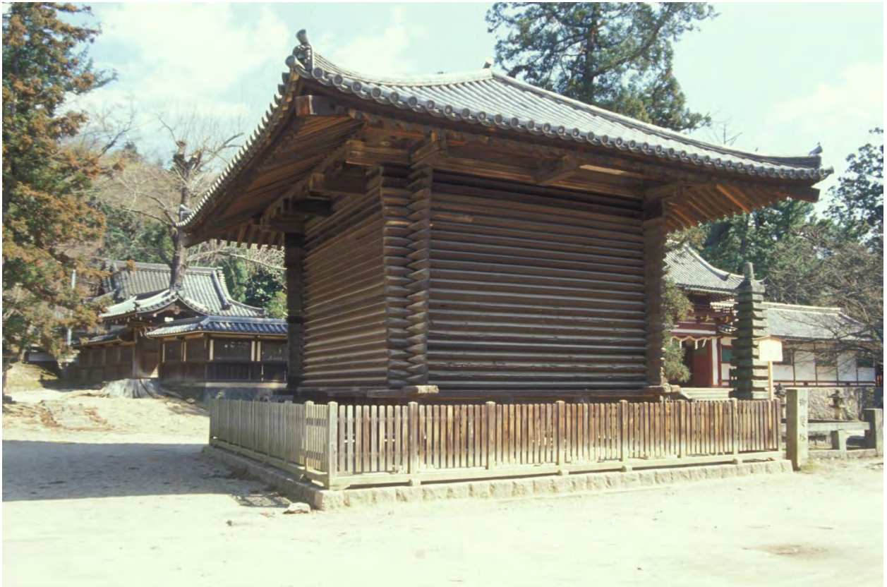
Figure 3.8 A log-structure from the Todai-ji Buddhist temple in Nara, Japan (Todai-ji Hokkedo Kyoko) This is the sutra repository, a storehouse for keeping the sacred books of Buddhism, built in the eighth century
