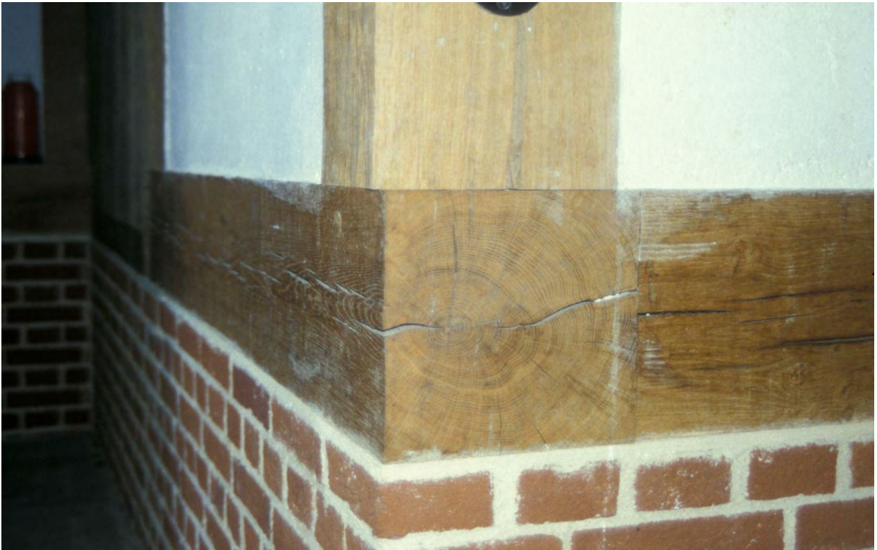
Figure 8.3 Shakespeare's Globe, London (1997). Oak heartwood ( Quercus robur ) was used in all external (exposed) members, although the architect and builder Peter McCurdy reckoned that the original structure probably contained timber with a high proportion of sapwood.
