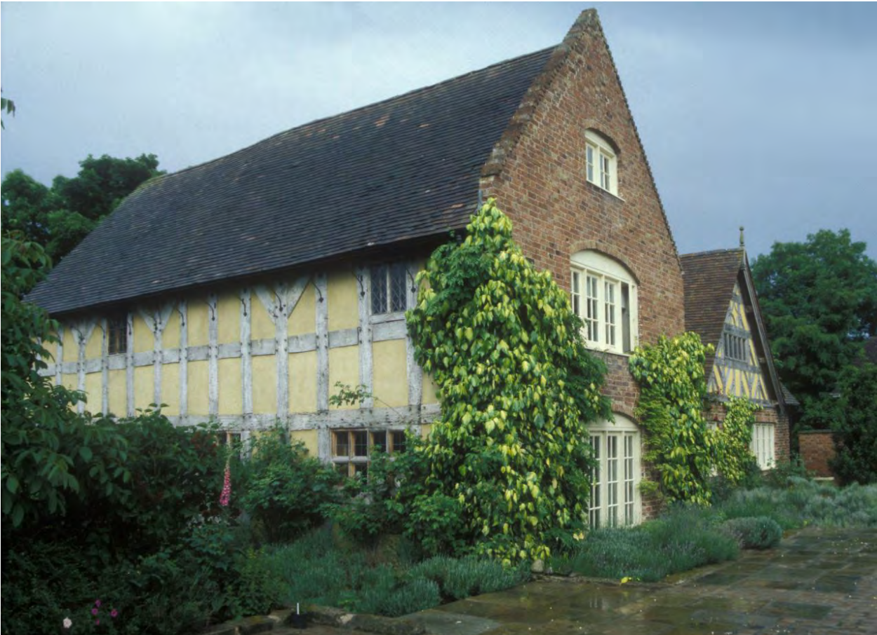
Figure 2.2 Brookgate Hall after restoration. Using the principle of minimum intervention, the architect conserved the timber structure and skilfully rebuilt the house to modern standards while retaining its historic atmosphere.
