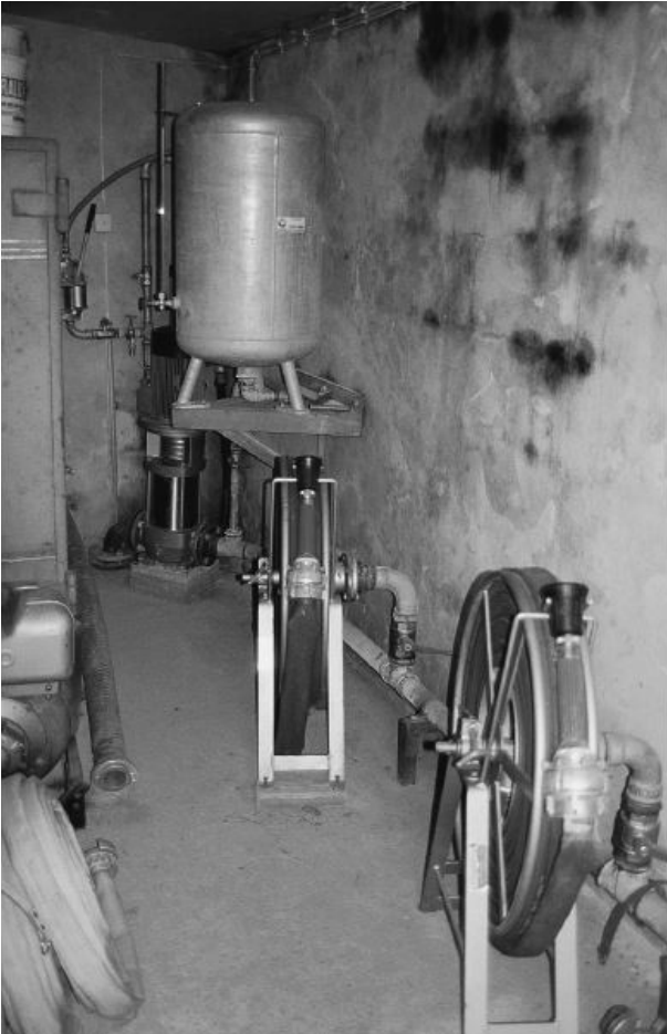
Figure 7.14 Fire protection equipment at a Norwegian farm where there are a number of listed buildings. The owner has created a small pond to provide water for the fire fighting equipment.
