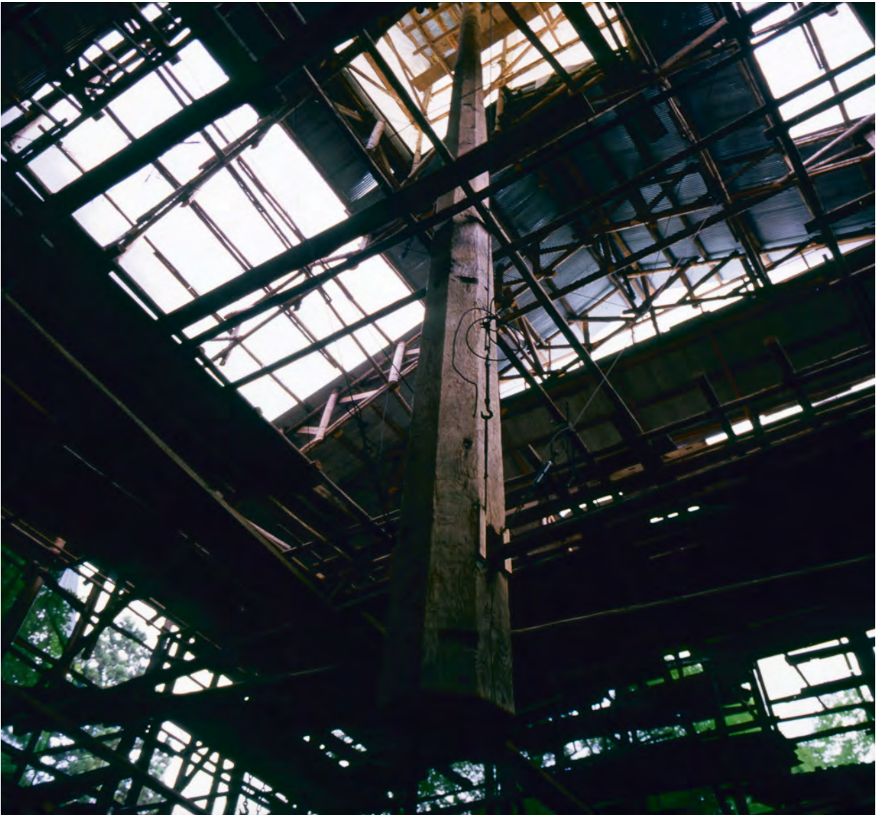
Figure 4.5 The central pillar of the three-storied Oyama-dera pagoda during preservation work in 1989. All members of the pagoda have been dismantled except the central pillar which is suspended from the scaffolding.
