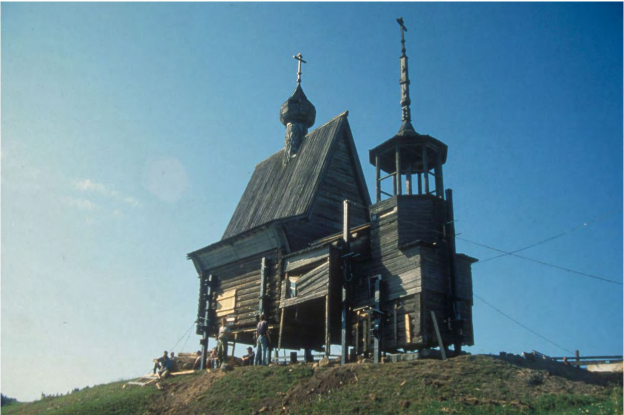
Figure 5.12 St. Nicolas Chapel, Kenozero National Park, Archangel, Russia, was restored in 1995-96 by Russian and Norwegian carpenters. The repair of the chapel is one of several joint Russian-Norwegian projects aimed at preservation of historic timber buildings through the revival of traditional techniques of craftsmanship. Hydraulic jacks and steel posts made it possible to renew rotten horizontal logs, while at the same time avoiding dismantling the chapel. (Photo by Anders Haslestad, Directorate for Cultural Heritage, Norway.)
