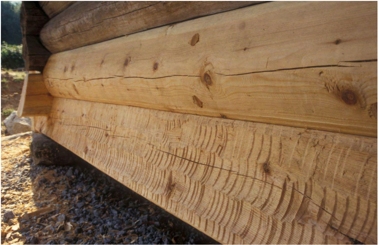
Figure 5.8 A sill beam prepared using sprett-telgjing .
