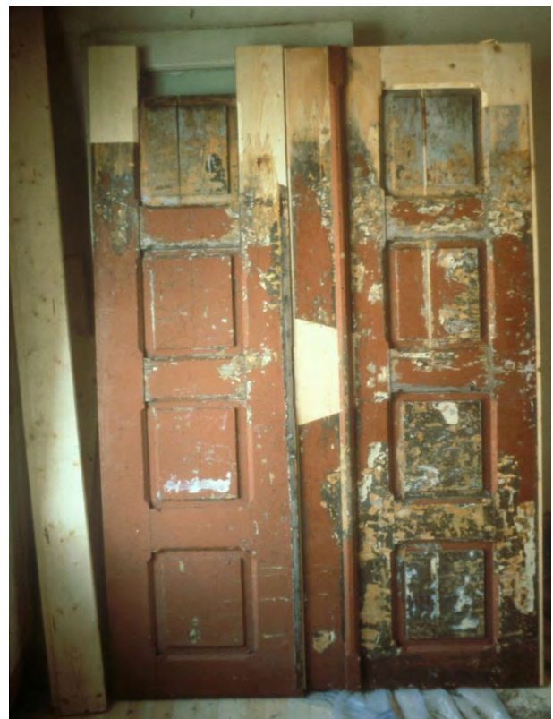
Figure 4.12 Pieced-in repair of a door. Mosjøen, Norway.
