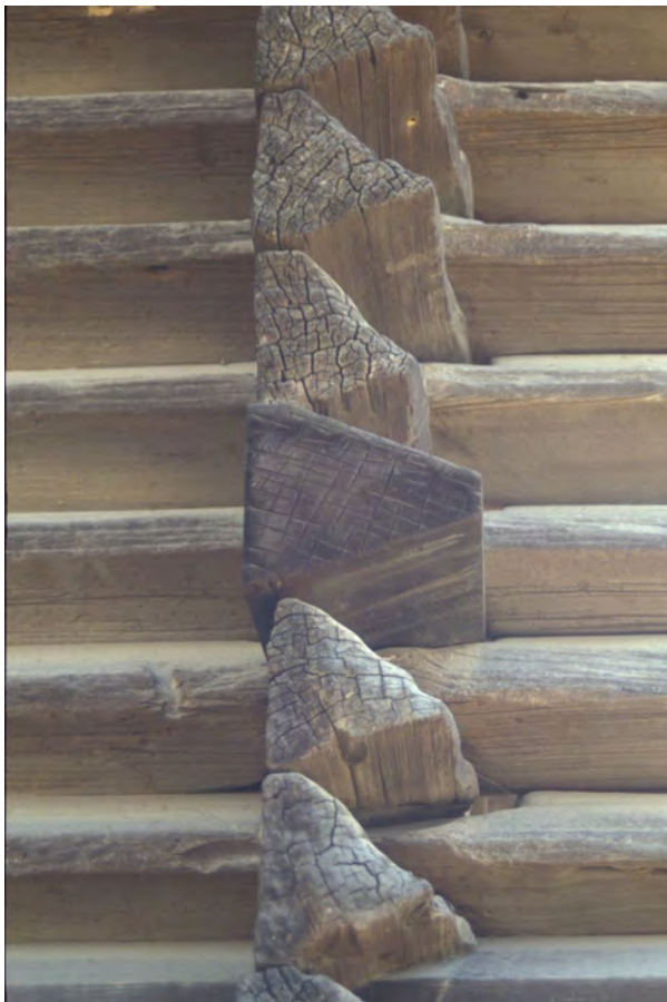
Figure 8.9 Detail from a log-structure from the Todai-ji temple in Nara, Japan, built in the eighth century (see Figure 3.8). The cross-section of the original eighth century logs has been greatly reduced due to weathering. The new log, clearly distinguishable, was added during repair completed in 1964.
