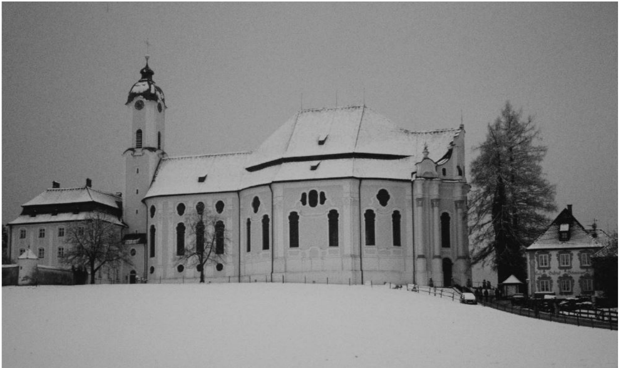
Figure 7.4 The pilgrimage church of Wies near Steingaden, Bavaria is a World Heritage site. It was built between 1745 and 1754. The church, situated in an alpine valley, is a masterpiece of rococo art and architecture. The masonry church walls and eight paired pillars carry a timbered roof structure and a wooden vault over the central area (the nave). The vault consists of ribs suspended in the roof structure, a construction typical of baroque churches. Laths are nailed to the ribs. The vault soffit is plastered and painted with beautiful frescoes. As the vault is linked to the roof structure, all forces affecting the roof, such as wind, consequently affect the vault and its stucco decorations.
