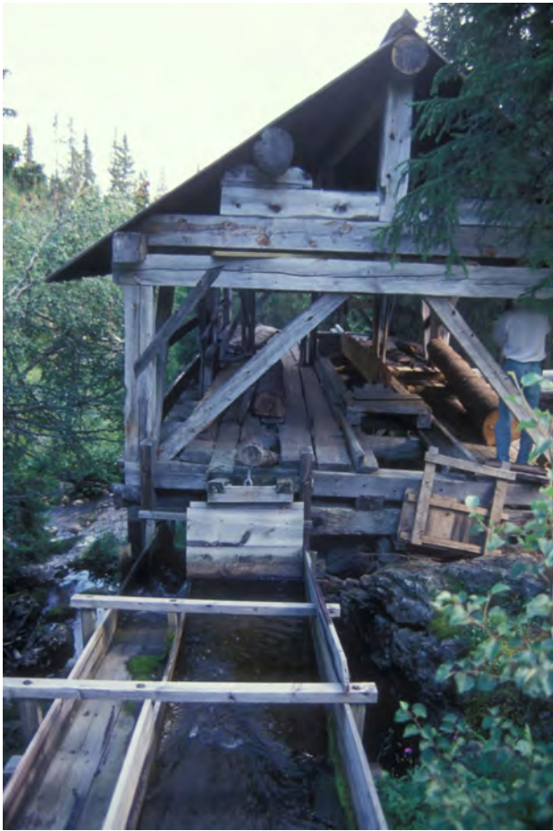
Figure 5.14 A frame saw in Rauland, Norway, which was restored together with the associated water-ways and dams as part of the Medieval Programme in Norway 1991-1996.
