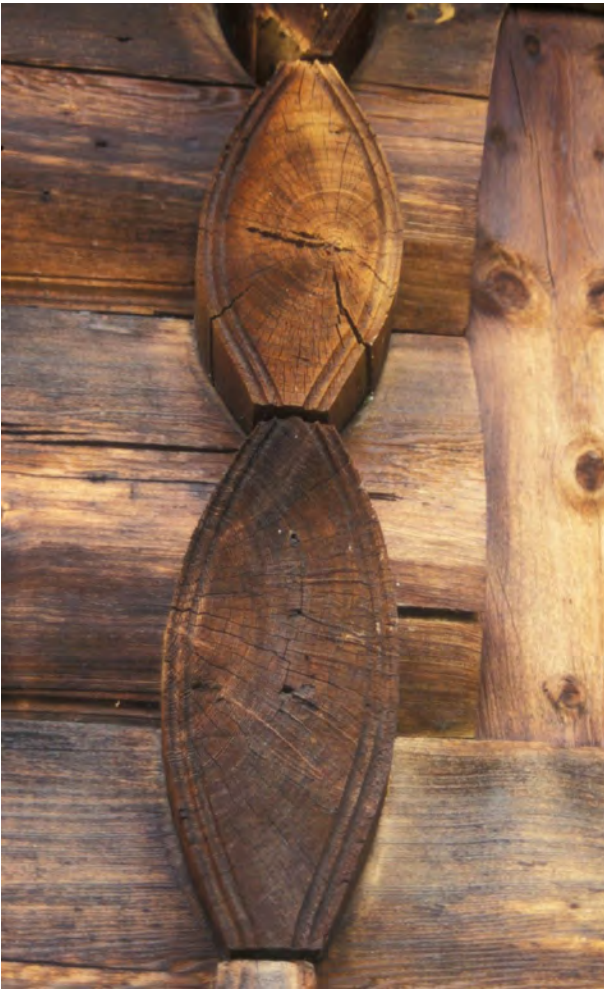
Figure 6.4 Detail of logs in a Norwegian log-structure from the late eighteenth century. Note the extremely narrow width of the annual rings
