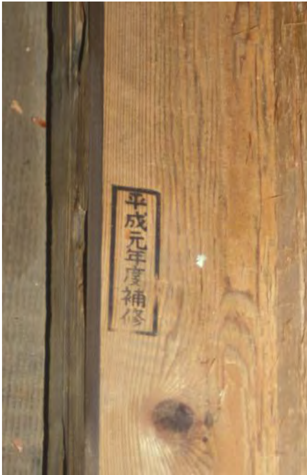
Figure 4.8 New members or parts of members should have the date of the repair inscribed on them so that they can be identified later. Here is an example from Japan where the date of the repair is burnt into the wood. The characters mean Heisei gannen go hoshu, that is: this piece of timber was put into the structure in 1989, the first year of the Heisei era.
