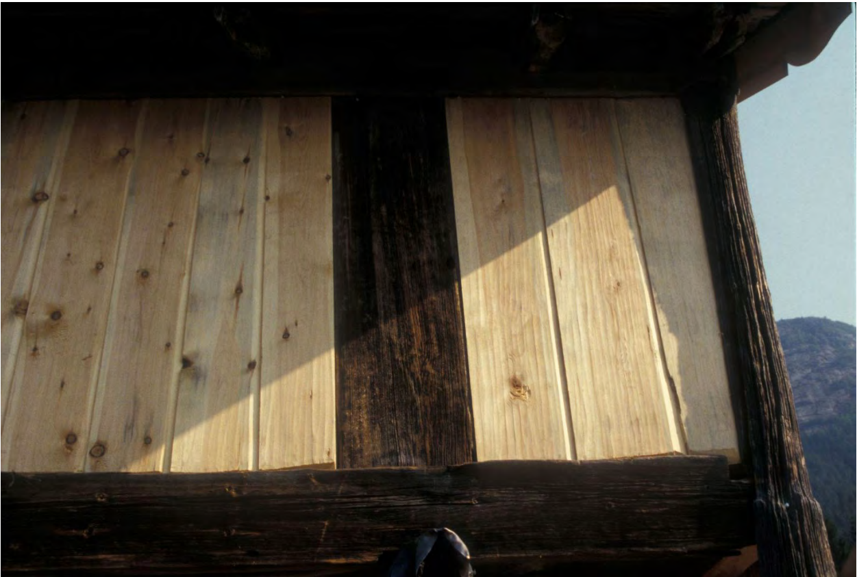
Figure 5.6 Boards inserted into the gallery wall of a Norwegian medieval timber structure during repair work. The boards have been planed using a spokeshave.
