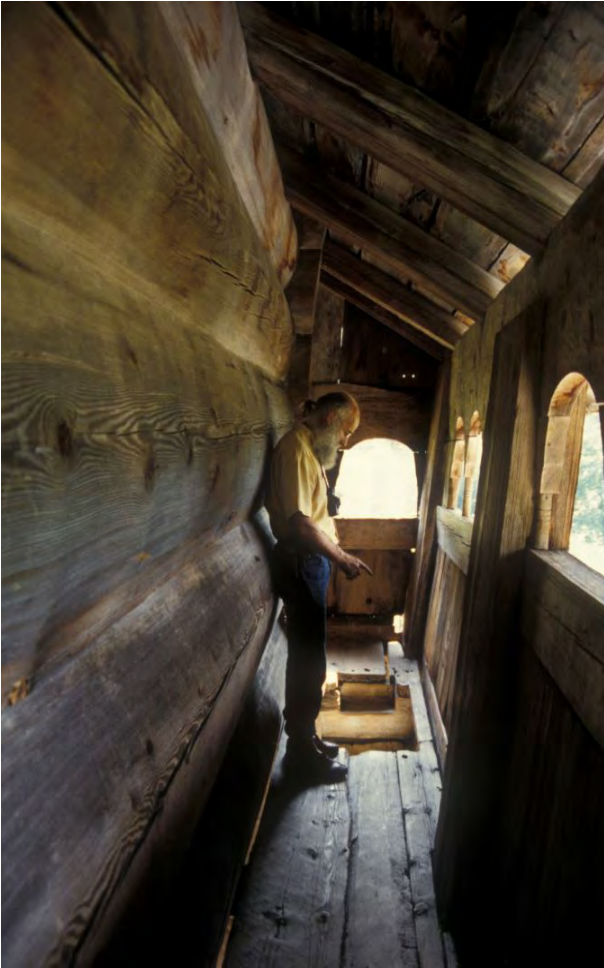
Figure 6.1 Large dimension timber from a late sixteenth century log-structure in Setesdal, Norway.
