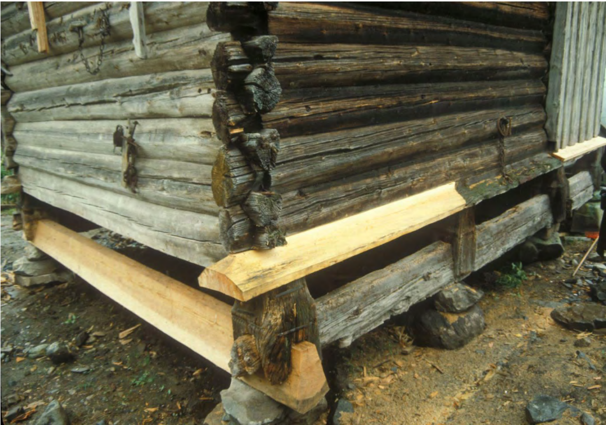
Figure 4.3 Repair in timber by copying old members. Tokke, Norway.
