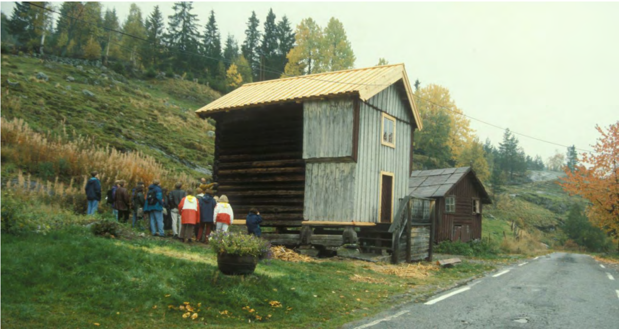
Figure 5.9 A repaired medieval timber building in Tokke, Norway. Only minor repairs have been made to the log-structure. The roof boarding has been completely renewed.
