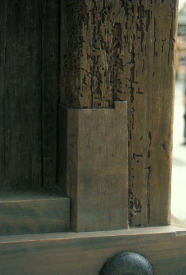
Figure 8.11 Detail of the Shakadō hall in the Kiyomizu-dera Buddhist temple, Kyoto, Japan, built in the eighteenth century. During the dismantling-repair process completed in 1975 the lower part of this corner pillar was repaired by jointing in new, well-seasoned timber. The new timber contrasts dramatically with the original timber, whose appearance is due to decay, insect attack and the effects of weathering.
