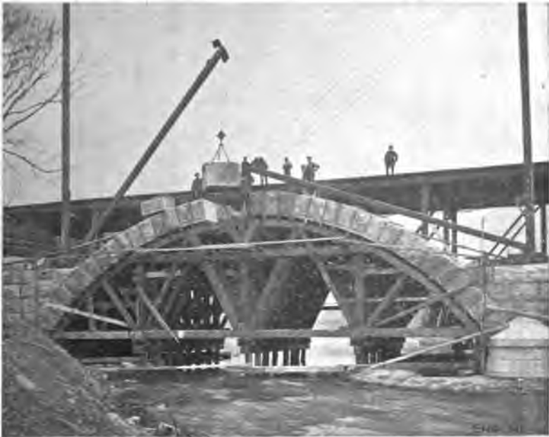
FIG. 75i. Stone Arch Bridge of C. M. & St. P. Ry., Watertown, Wis.
