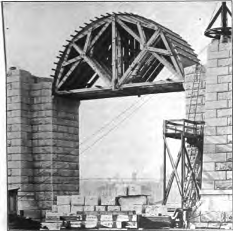
FIG. 75 k . Center for Pier Arch of Queensboro Bridge, New York.
